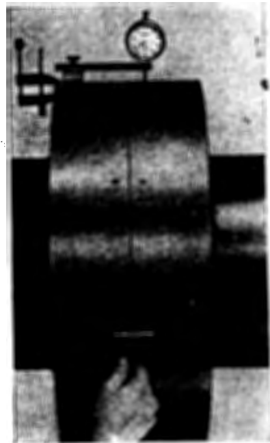
Fig. 2.15b Checking the radial alignment with dial gauge
